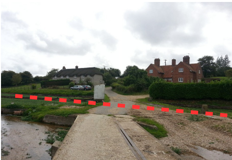
Level Crossing on Hollow Oak (break point between north and south systems)
